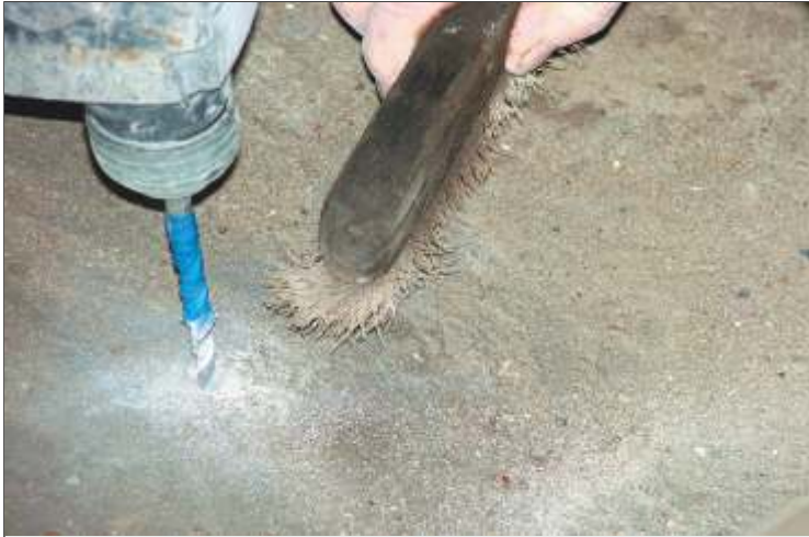
Hand using a brush to clean the concrete surface.
