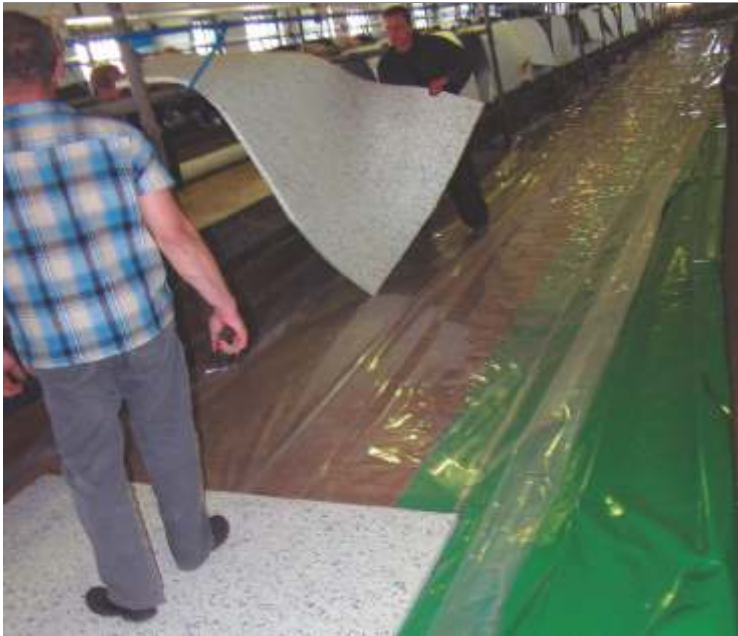
Workers handling a large sheet of material over the waterproofing membrane.
